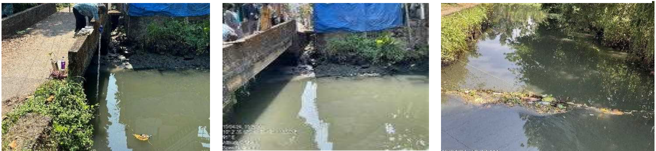
Plate 3: Edappally Canal (EC-01) at 30 m downstream of the confluence of the Periyar River and Edappally Canal (Lat.: 10° 2'36." and Long.: 76°18'12." )
