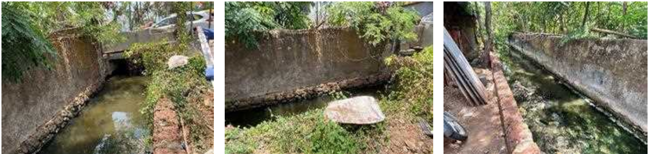
Plate 14: Valiyath Canal (VC-01) located at 0.1 km upstream of the Pallikal River (Lat.: 9° 3'25.04" and Long.: 76°32'30.56")
