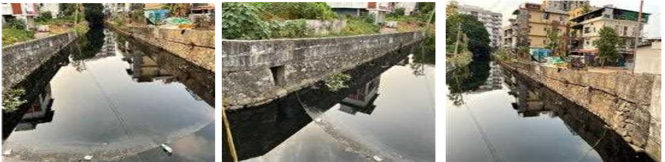
Plate 8: Thevara-Perandoor (TPC-03) Located at 3.25 km downstream of TPC-02 near Gokulam Convention Centre (Lat.: 9°59'43" and Long.:76°17'24")
