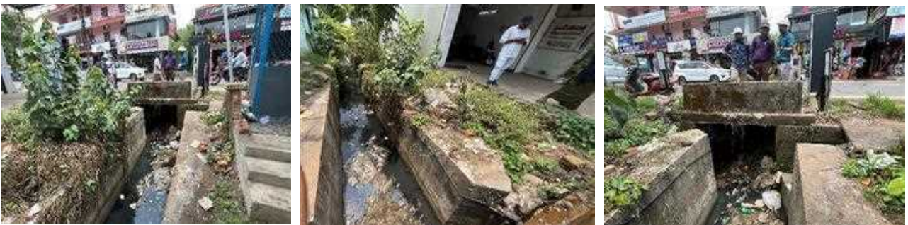
Plate 19: Valiyath Canal (VC-06) located at 3.0 km upstream of the Pallikal River (Lat.: 9° 4'38.76" and Long.: 76°32'2.30")
